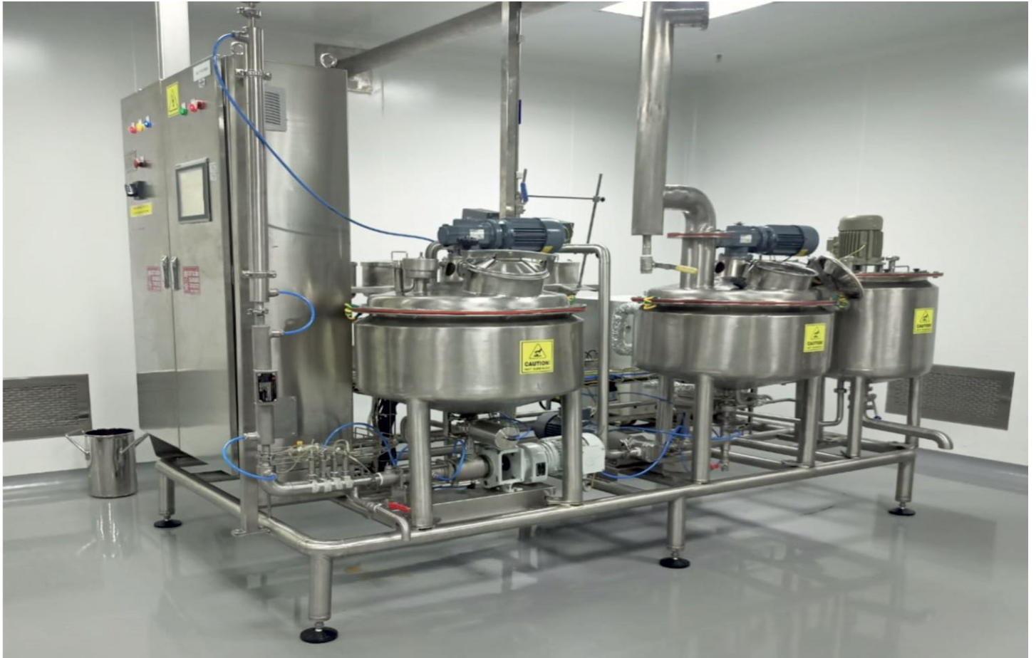
BAR LINE UNIT
